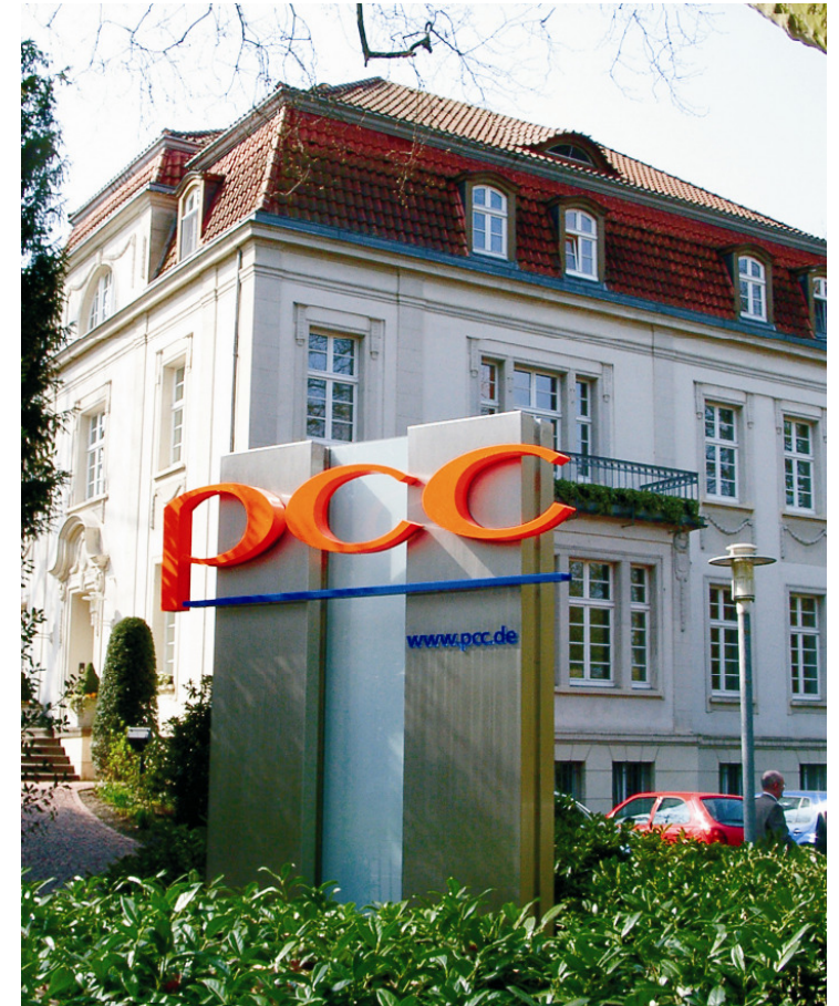
PCC Headquarters in Duisburg (Germany)
